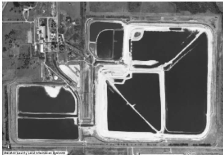
Four ponds are located on top of the Piney Point gypsum stacks with a series of smaller ponds located on the west side.
