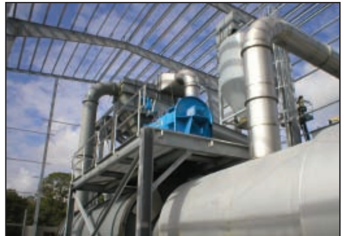
The roof to the new dryer facility under construction
