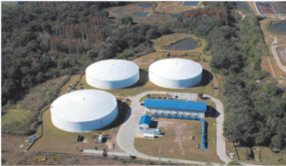
Figure 6: High Service Pump Station
