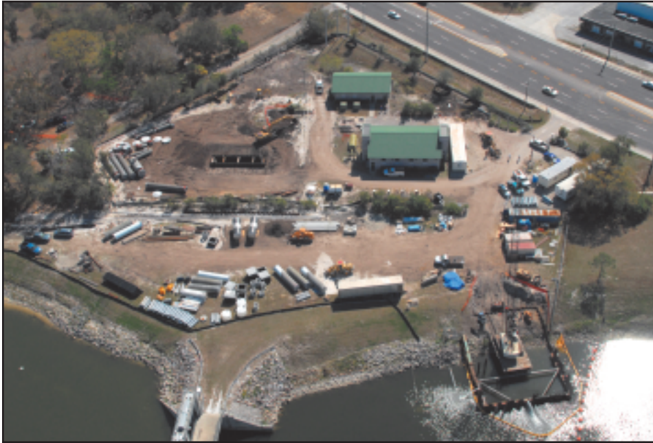
Figure 3: Aerial View, Tampa Bypass Canal Pump Station Expansion Site
