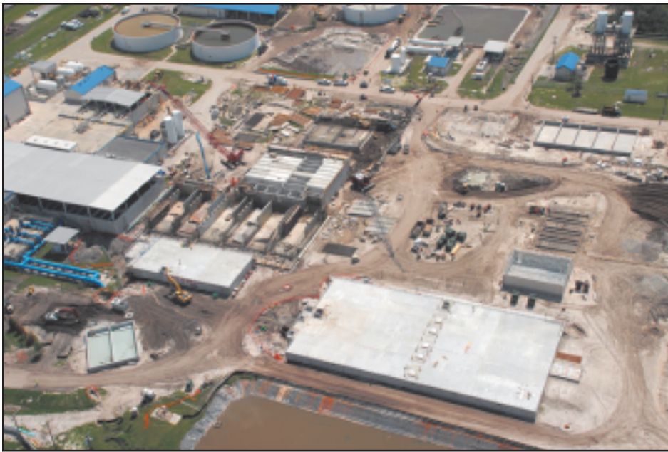
Figure 18: Surface Water Treatment Plant Expansion Construction
