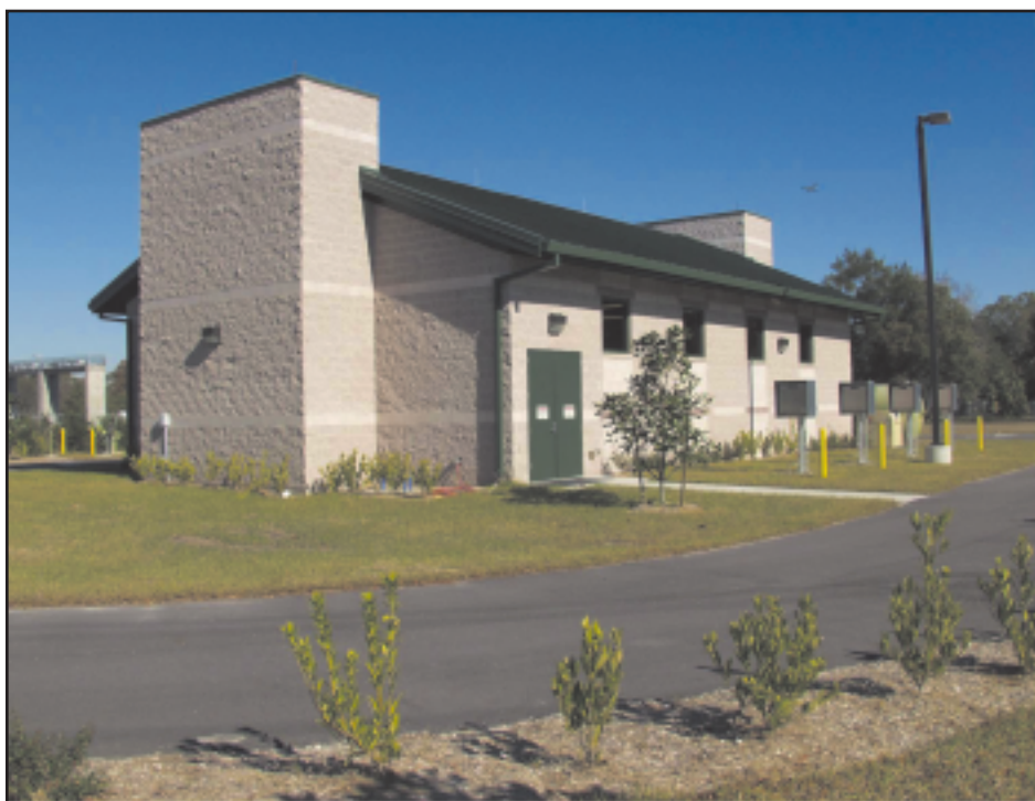
Figure 2: Tampa Bypass Canal Pump Station
