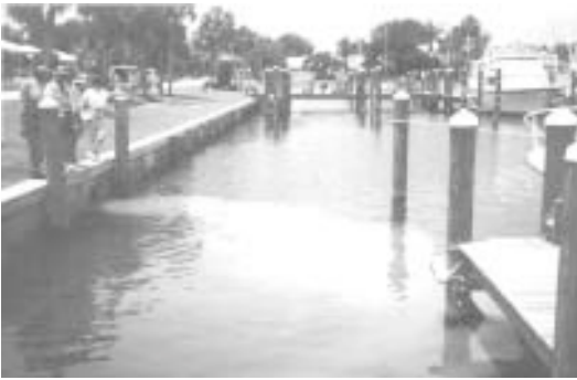
Figure 1. Dyed effluent entering the boat basin from the storm sewer.
