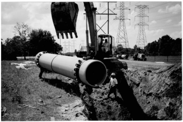
Service Area WWTF. Because many of the existing smaller pump stations were having to pump against heads that exceeded design heads, the county needed a new force main so that flows from the Conway Master Pump Station could be diverted from the existing system, allowing the existing pump stations to operate within their design conditions.
