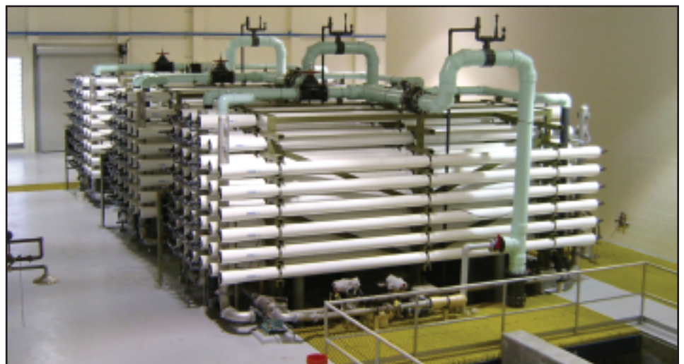
Three 2-MGD reverse-osmosis skids provide treatment of the brackish raw water from the Floridan Aquifer.
