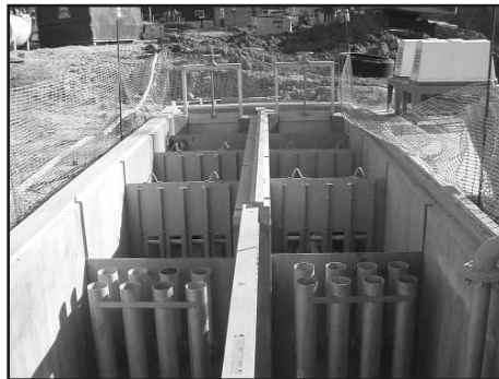
Figure 7. UltraGuard LP-HO system Courtesy of UltraGuard as subsidiary of US Filter
